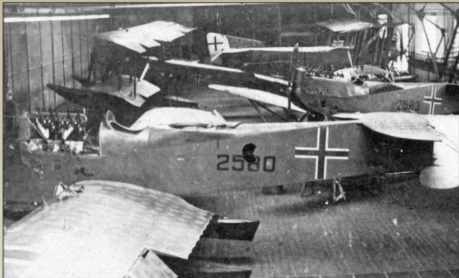
C2MGHFT W.29s 2580 and 2583 await demolition at Wilhelmshaven after the armistice. Both aircraft were from a batch of 20 C2MGHFT W.29s (numbers 2564 to 2583) ordered in late May 1918 and feature late production tailplanes (89). The anemometer has been removed from 2580 and neither aircraft has any weapons fitted. What appears to be a hole in the side of 2580 is damage to the photograph negative.
