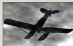
^ This dramatic bottom view of an unidentified W.29 allows us to see the modified tailplane. The tips of the horizontal tailplane have been cut off but it retains the production elevators.
