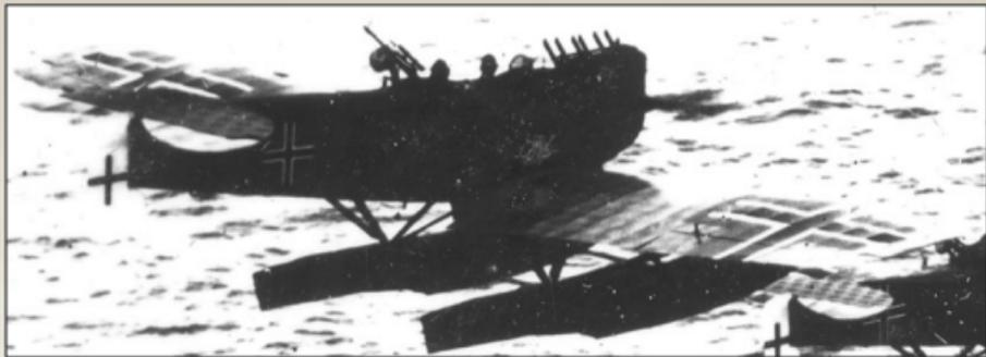
W.29 22?? (the full number is not legible) showing how the March 1918 balkenkruetz design has been converted to the thinner style introduced at the end of June by overpainting the earlier style with black and white and grey paint. On this particular aircraft the June balkenkruetz have been painted slightly outboard of the earlier ones, but this was not always the case. Note the 2-2-2 arrangement of the Benz Bz.III exhaust and Parabellum LMG 14/18 with Oigee optical sight.
